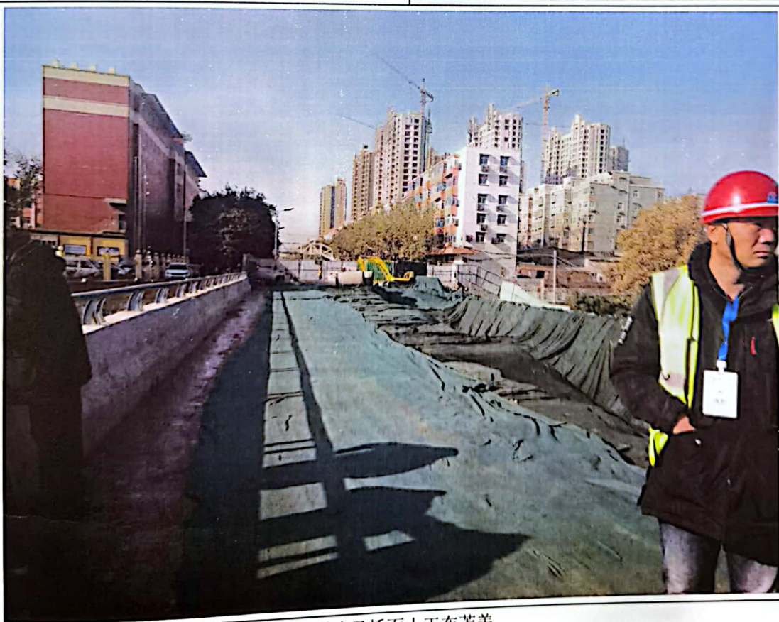
桥头及桥面土工布苫盖
